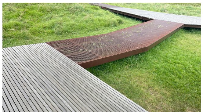
Figure 95: Materiality of timber and steel at Maungawhau Tihi Boardwalk. Author's own image.
