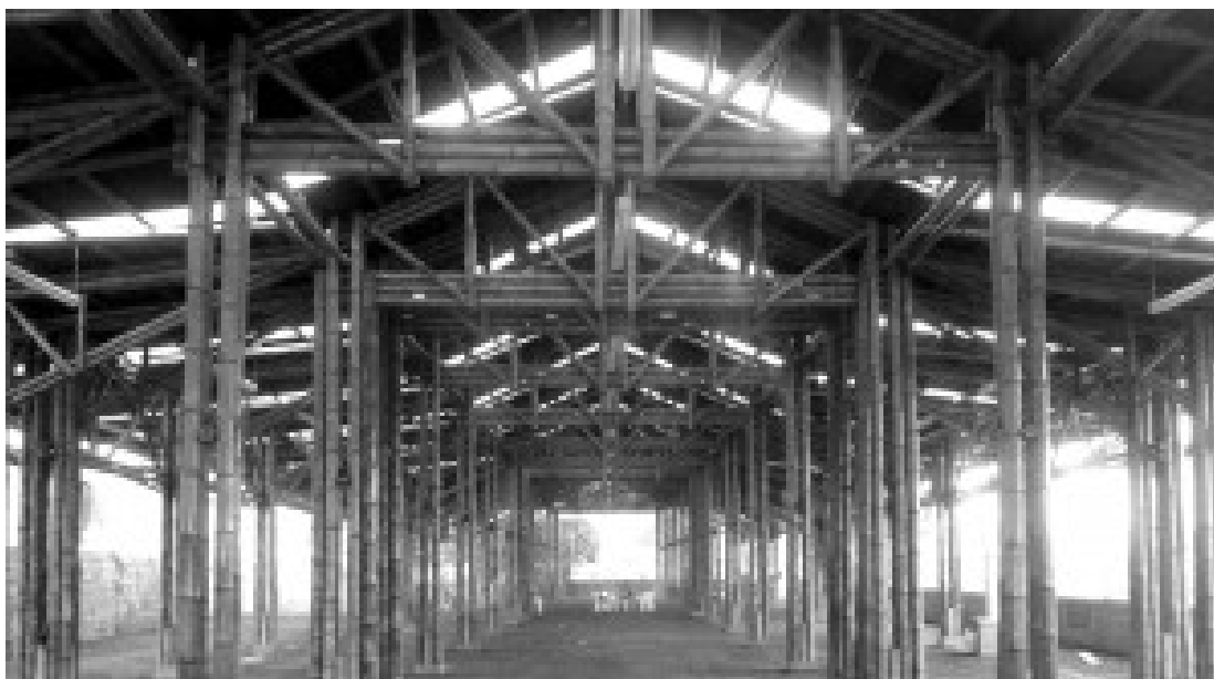
Figure caption: A 2,000m 2 warehouse using Guadua in Bogotá DC, Colombia. All images credited to: Hector Archila.
