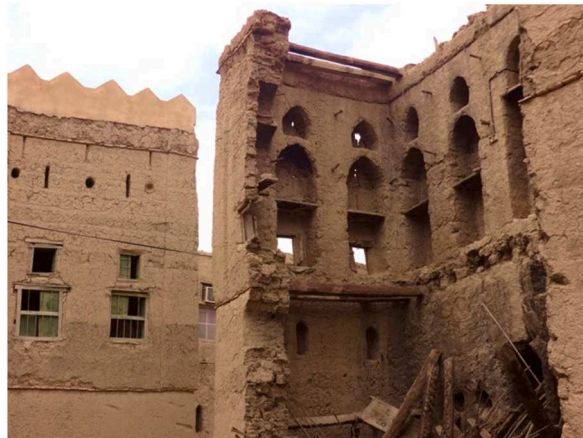
Fig 4. Omani heritage house built with Sarooj, wadi stones, and date palm trunks. Picture attribute Bait Al Safah Museum.
