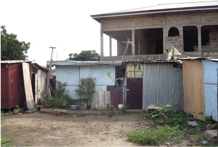
Fig. 3 Kiosks made out of wood sheets and corrugated iron roofs in Edano. Source: Authors, 2017
