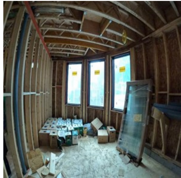
Picture 1. Bachelor room in a social housing building under construction
