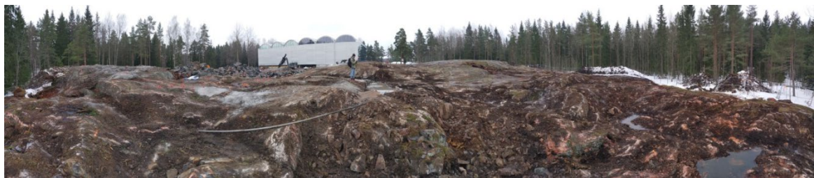
The construction site in Pirkkola, March 2021.
