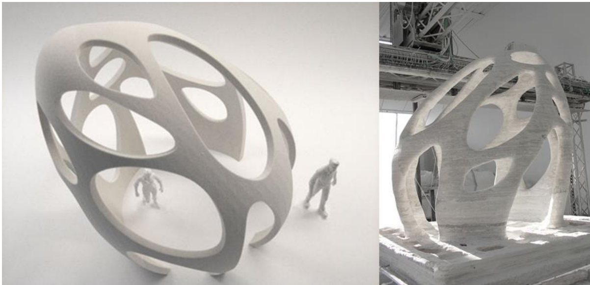
Figure 8. The Radiolaria pavilion by Andrea Morgante, a complex, free-form structure produced by additive manufacturing. https://www.dezeen.com/2009/06/22/radiolaria-pavilion-by-shiro-studio/ .
