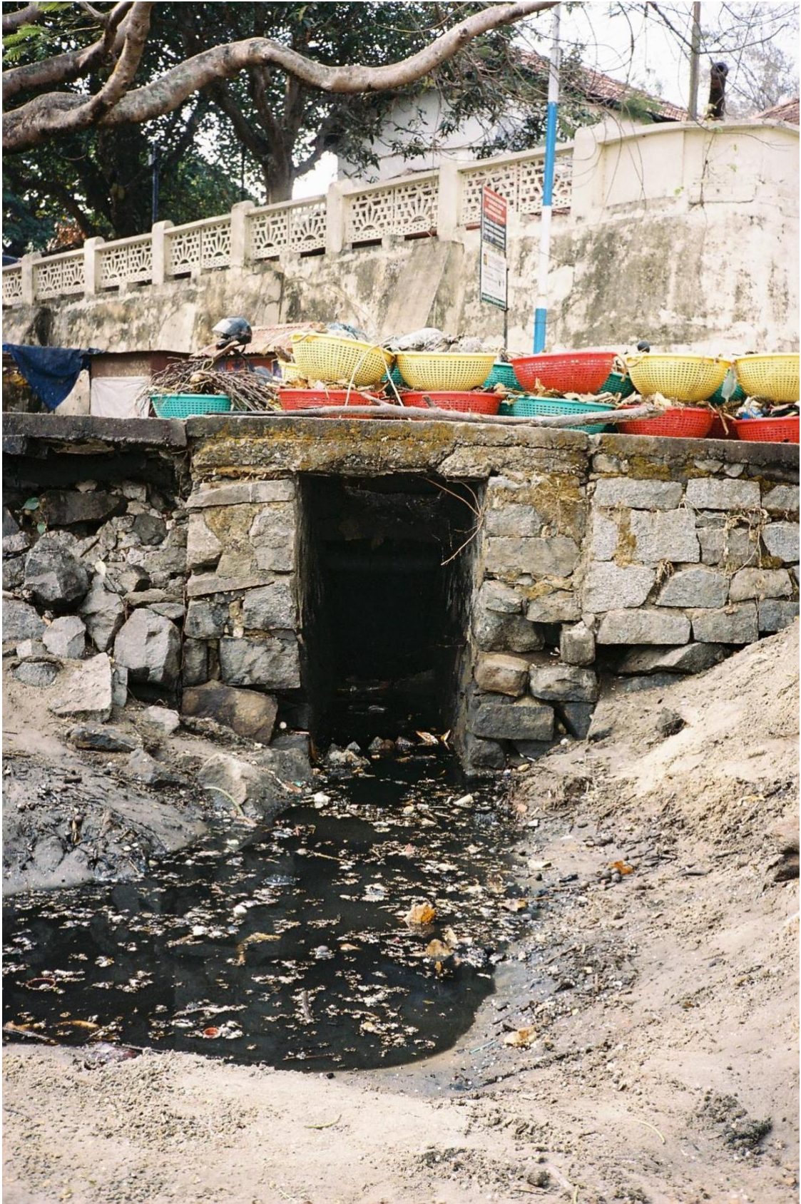
Figure 26: British era sewer, Mahatma Gandhi Beach. Fort Kochi.
