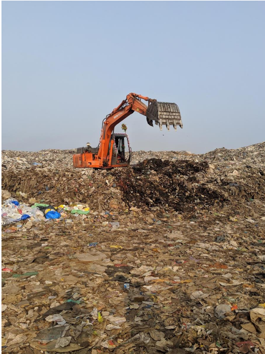
Figure 13: Decorated excavator moving legacy waste.
