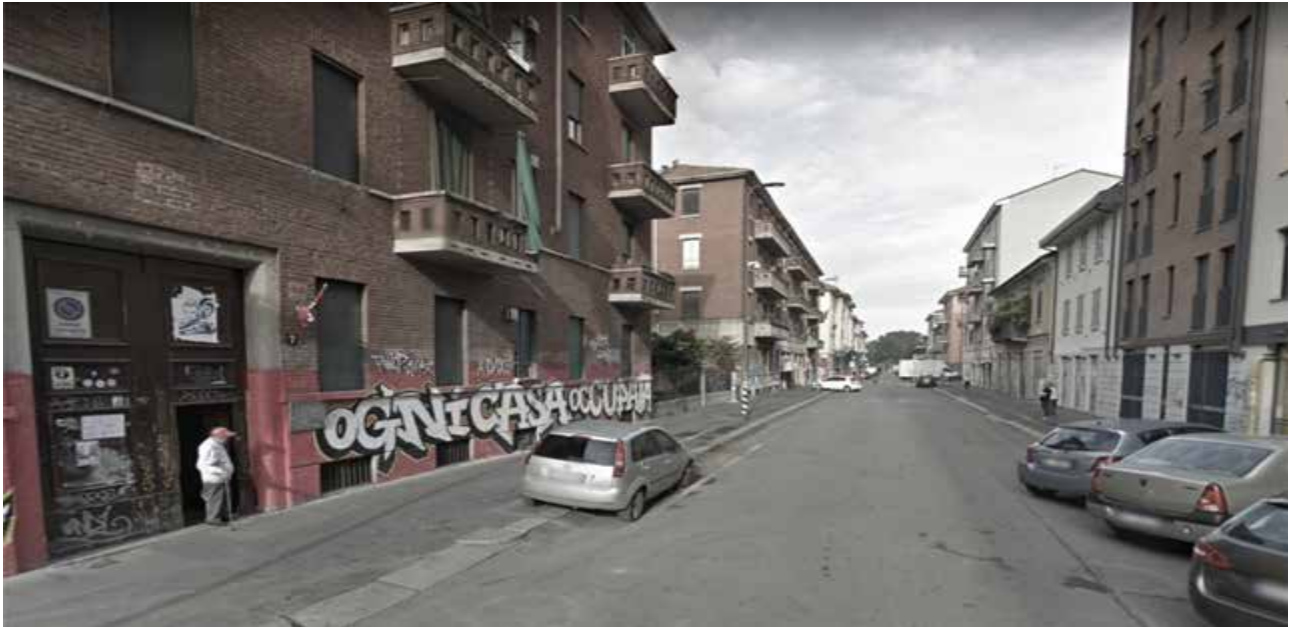
Figure 13. Current appearance of Via Emilio Gola, Milan (Italy): a desert, asphalted street, that causes feeling of discomfort and unsafety while crossing it. Photo credits: Google Maps.
