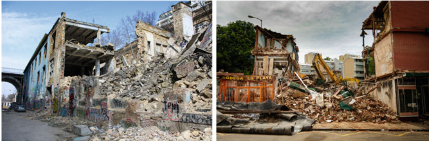
Fig. 1 Examples of urban masonry buildings damaged by earthquakes
