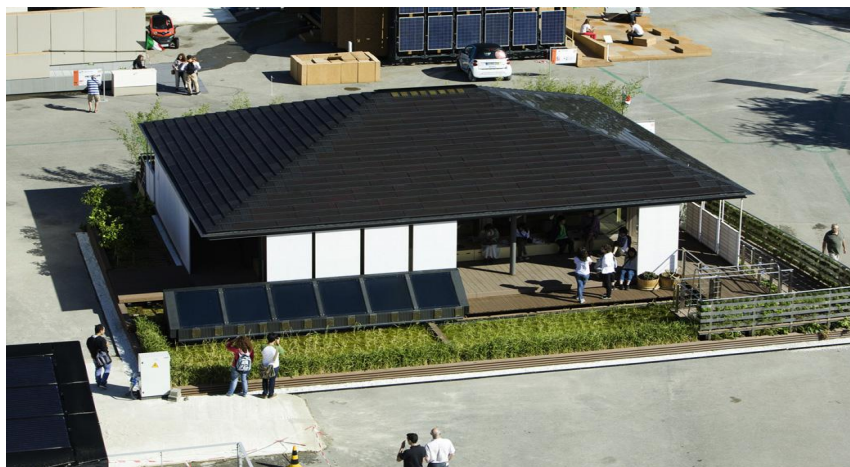
Figure 3: Roof Integrated BIPV System [38]
