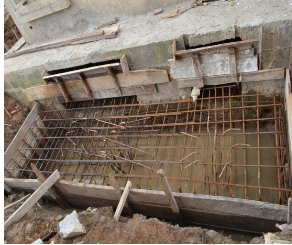
Fig. 17. Laid Beam anchored to underpinning piles
