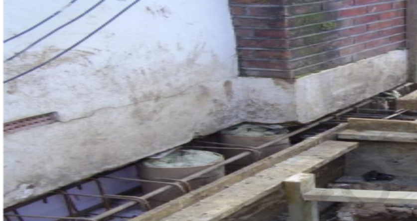
Fig. 7. Piles and Beams to support vertical loads [2].
