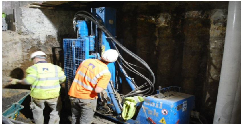
Fig. 6. Mini piling underpinning to support vertical loads [2].
