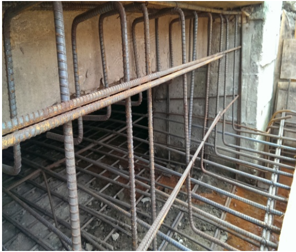
Fig. 16. Laid reinforcement cages
