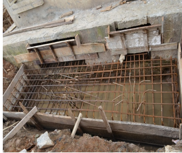
Fig. 17. Laid Beam anchored to underpinning piles
