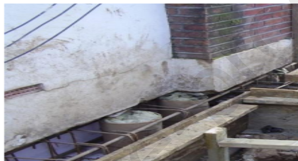
Fig. 7 Piles and Beams to support vertical loads [2].
