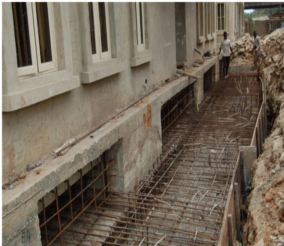
Fig. 18. Laid Beam anchored to existing raft
