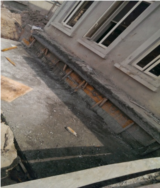
Fig. 22. Completed underpinning work.
