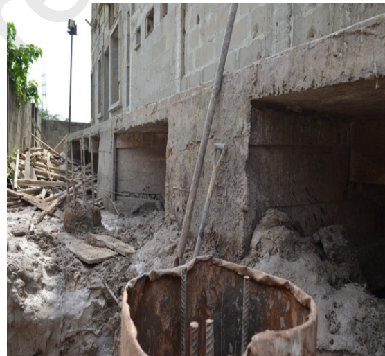
Fig. 15. Bored piles for underpinning
