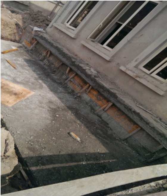
Fig. 22. Completed underpinning work.
