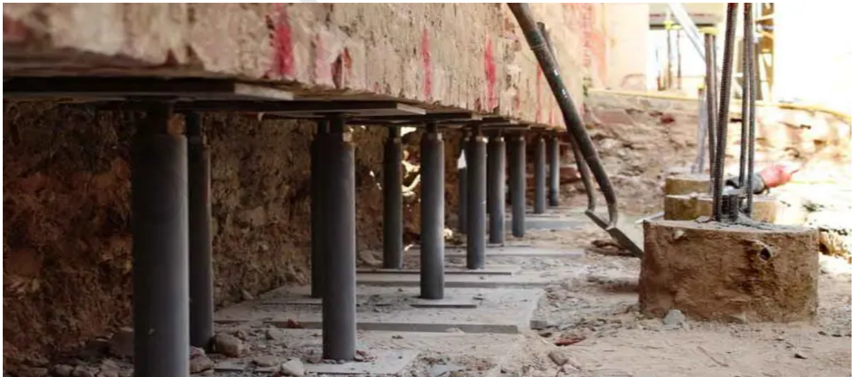
Fig. 2. Pynford stool for underpinning [35].
