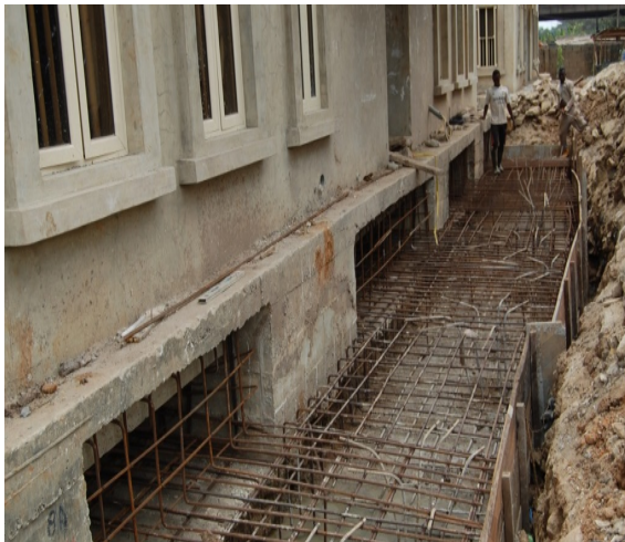
Fig. 18. Laid Beam anchored to existing raft
