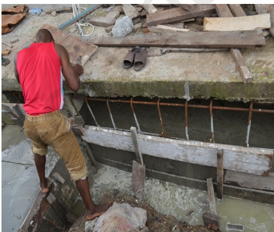
Fig. 20. Shuttering work
