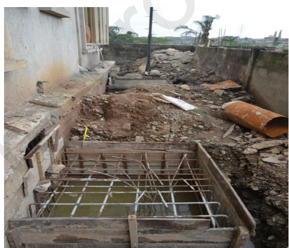
Fig. 19. Pile cap with ground beams
