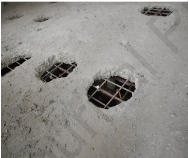
Fig. 14. Opening of holes in the veranda slab
