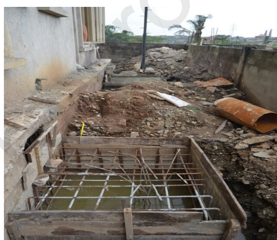
Fig. 19. Pile cap with ground beams
