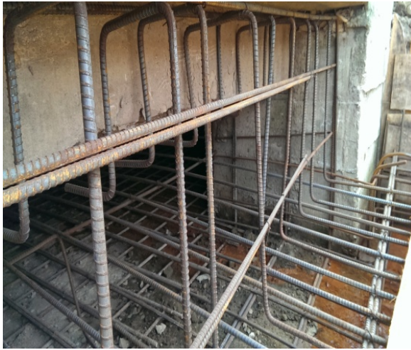
Fig. 16. Laid reinforcement cages
