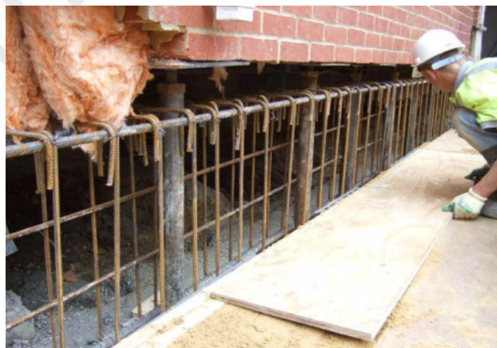
Fig. 4. Beam and Column underpinning [32].
