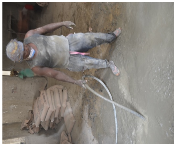
Fig. 21. Use of Poker vibrator
