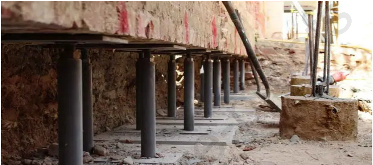
Fig. 2. Pynford stool for underpinning [35]
