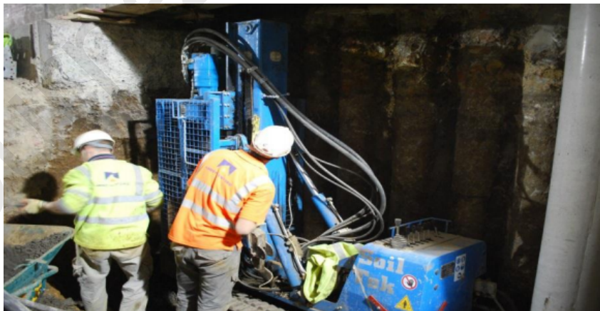
Fig. 6. Mini piling underpinning to support vertical loads [2].
