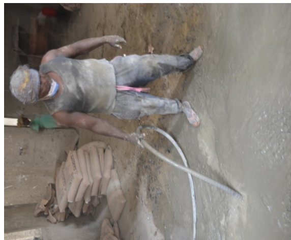
Fig. 21. Use of Poker vibrator
