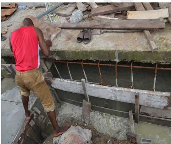
Fig. 20. Shuttering work
