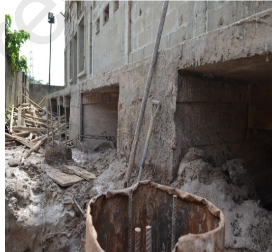
Fig. 15. Bored piles for underpinning
