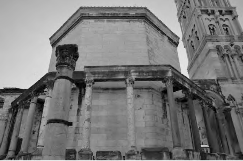
14a Split, Diokletiansmausoleum
