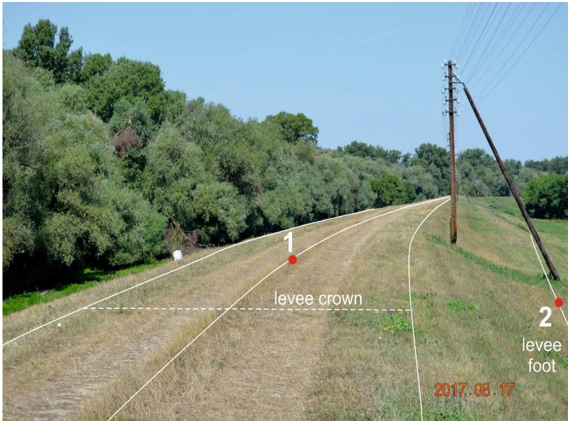
Figure 3 Location of GPS points measured on levee crown and levee foot
