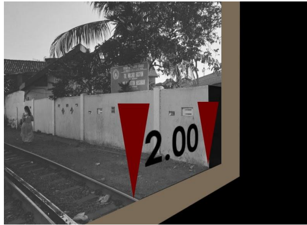
FIGURE 2. The Distance Between the Train Tracks And Uswatun Hasanah Elementary School Surabaya
