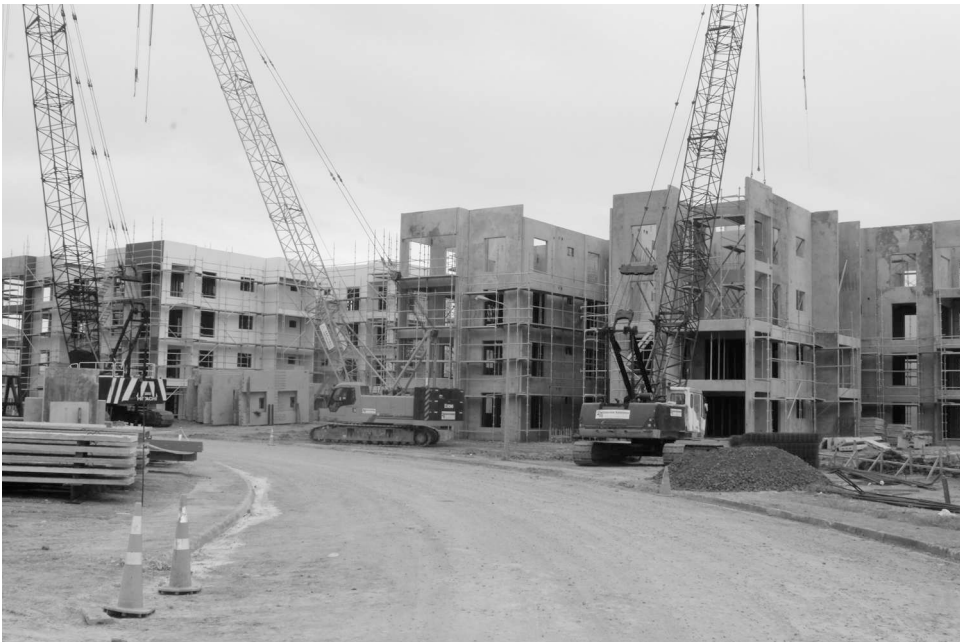
Figure 26.3 Construction of luxury apartments some 200 m from Muanivatu (Weber; Feb. 2021).
