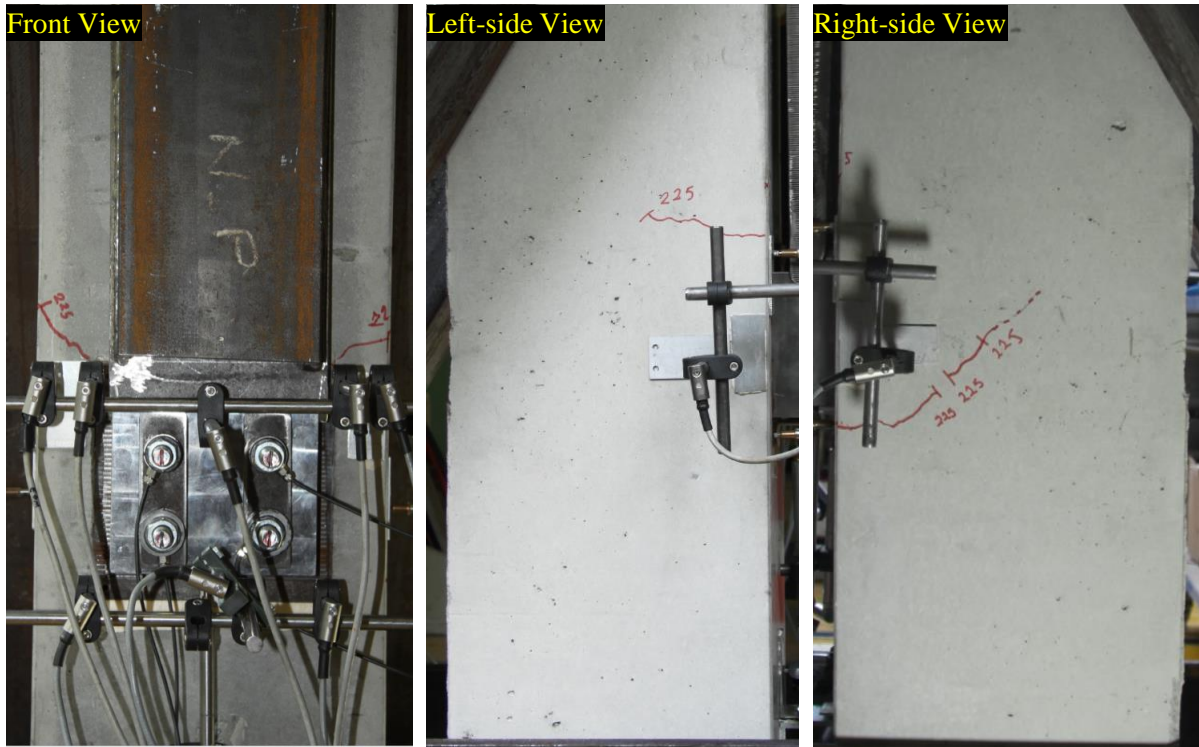
Figure 3.44: Crack patterns at 225kN (60% of F_{u,exp} ) / CC-01.
