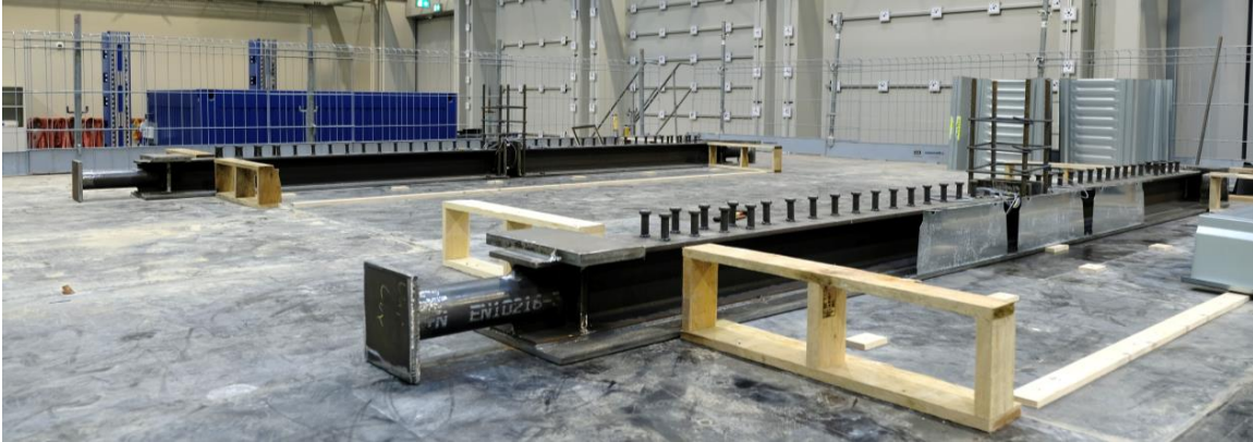
Positioning of Steel Metal Sheeting
