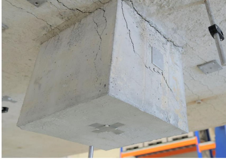
Figure 5.21: Tensile crack formation for GJSFB-01 test specimen.
