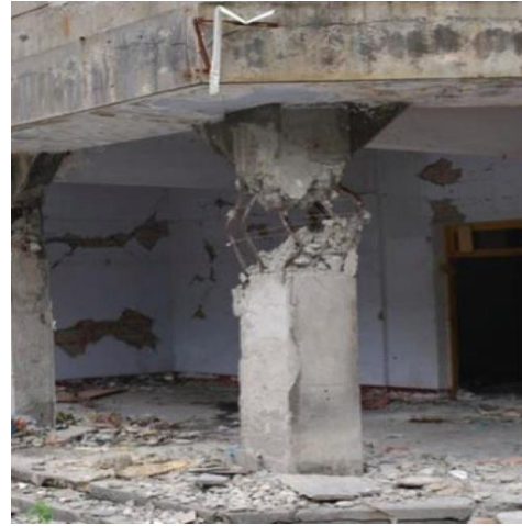
(e) Building Column Hinging at Base and Top (6)
