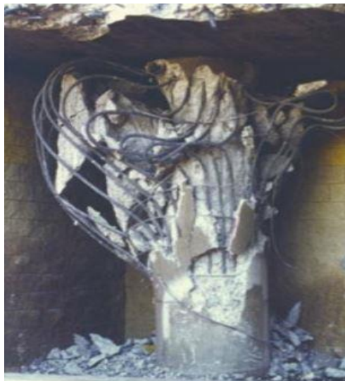
(g) Lack of confinement reinforcement (6)
