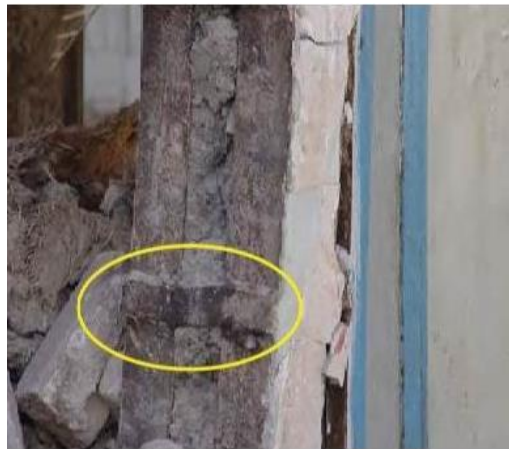
Plastic deformation of battens
