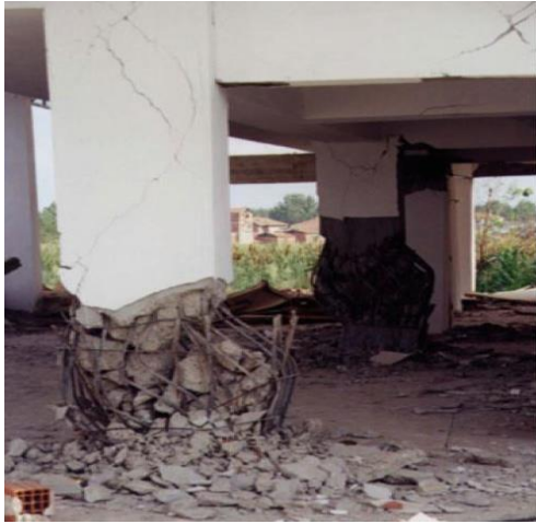
(e) Building Column Hinging at Base and Top (6)
