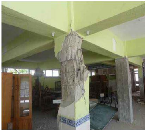
(f) Collapse of Buildings due to Strong Beam-weak Columns (6)(7)
