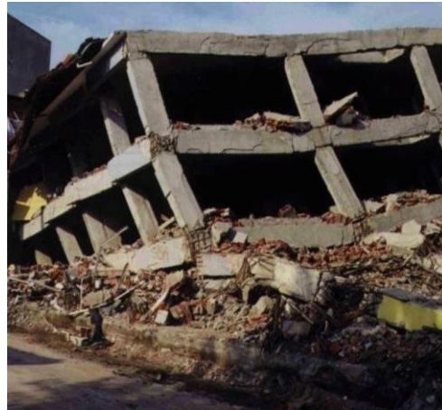
(f) Collapse of Buildings due to Strong Beam-weak Columns (6)(7)
