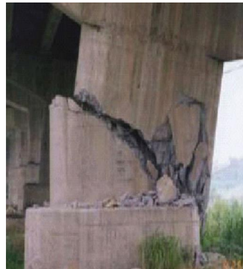
(h) Shear failure of Bridge Columns (6)
