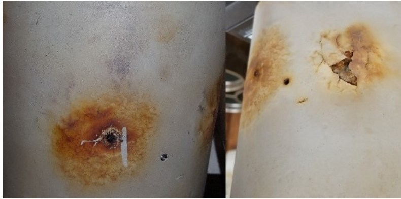
Figure 4.12: Pipe 17 showing July (left) and December (right) surfaces near instrumentation.
