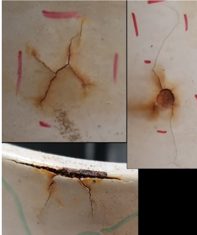
Figure 3.9: Pipe 13, Cracks in coating. Top right further examined in Figure 3.11.
