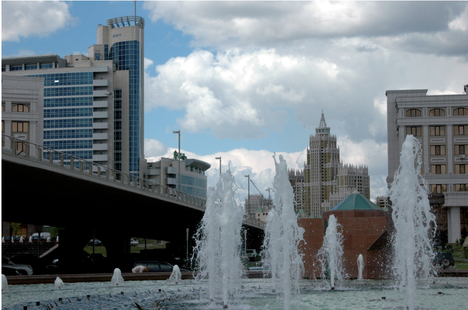
Figure 3. "Moscow"-style building in Astana, photo: by Author
