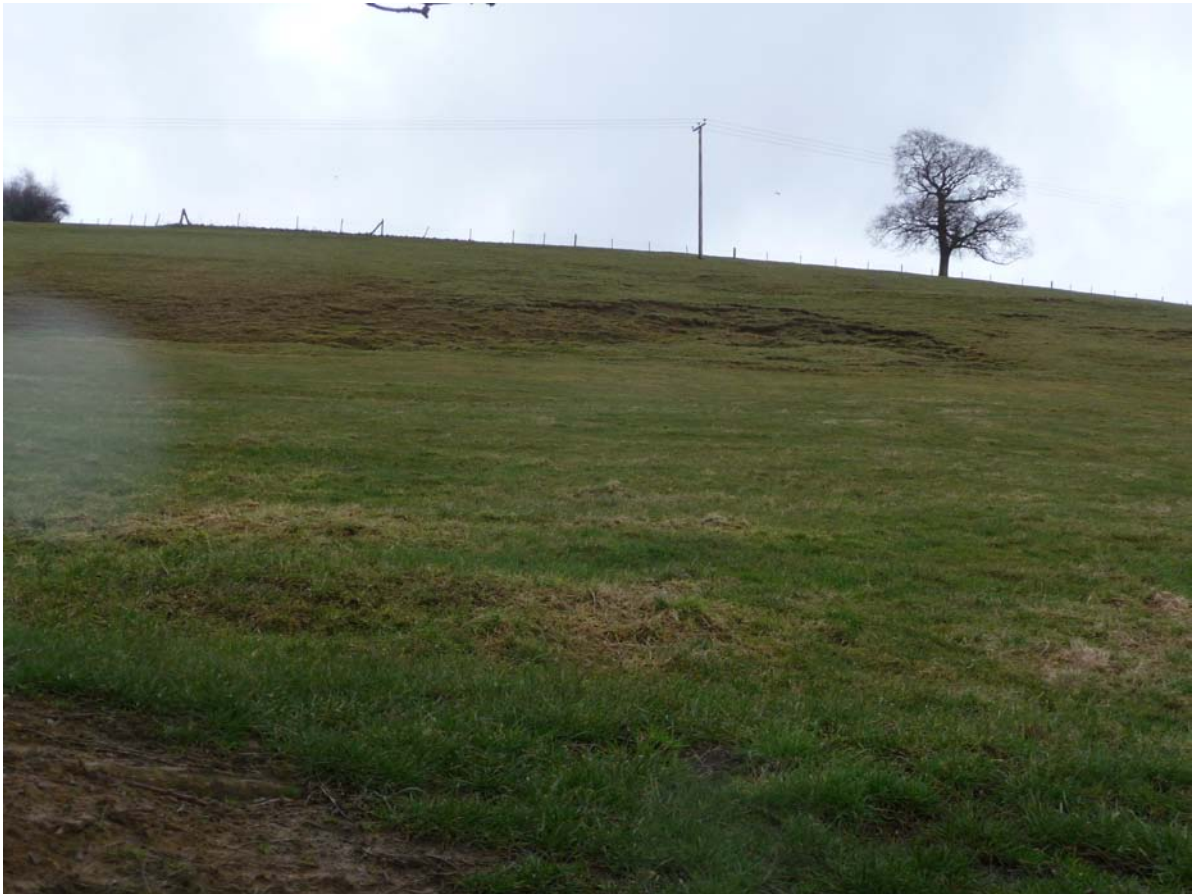
Figure 5. Fresh scarp features within the Mill House landslide. Photograph taken from NGR 495797 375113, orientation 090°.
