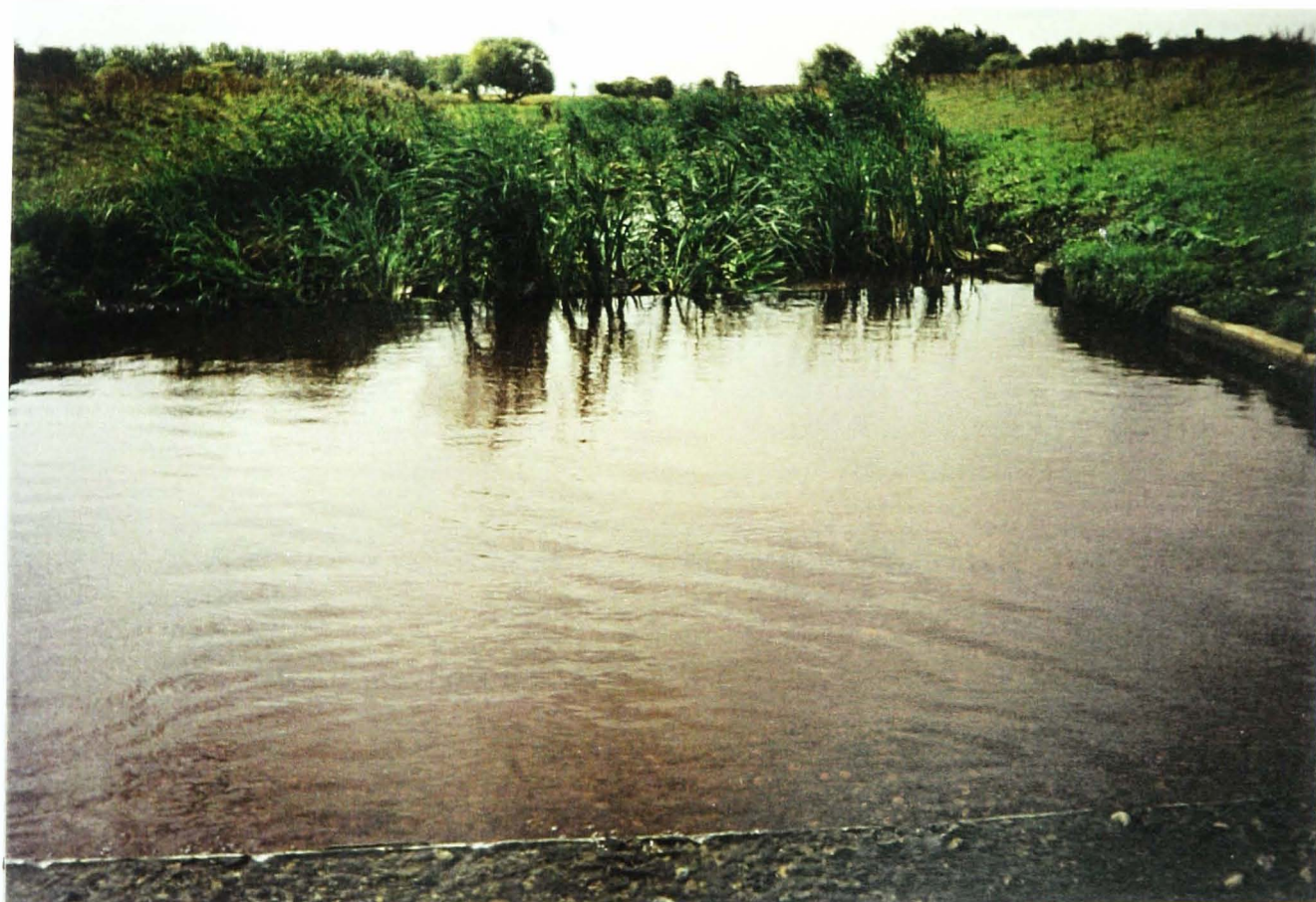
Figure 3. 5 View looking downstream across the settlement tank and the start of bed 1 (planted with Typha latifolia )
