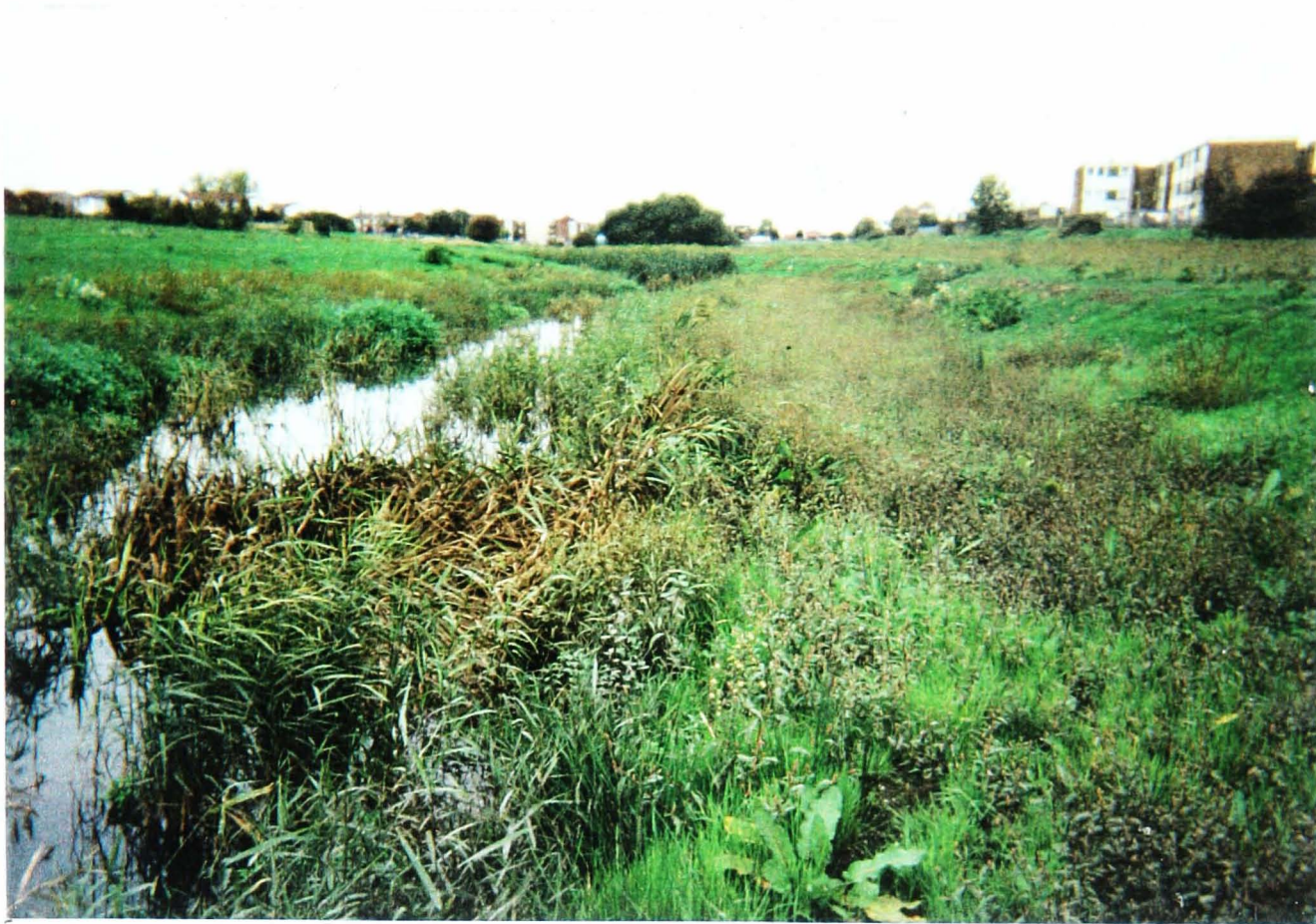
Figure 3. 6 View along wetland system looking up through bed 2 (planted with Phragmites australis ) up to end of bed 1 (planted with Typha latifolia ).
