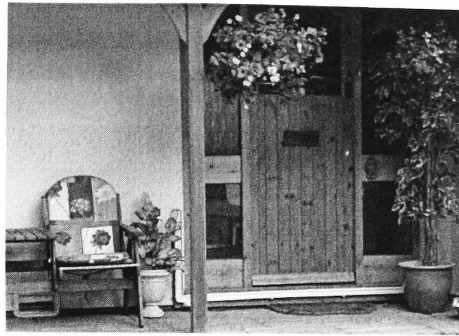
Back frame in place for flood guard and air brick.
