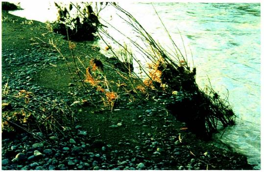
Photo 6.10. Siltation baffle resisting lateral erosion caused by thalweg migrationduring flood recession, 14 Jan 1995.
