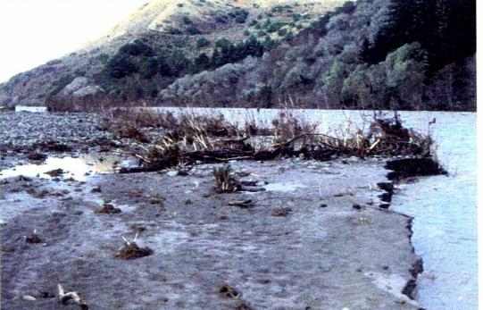
Photo 6.8. Scour beneath root zone of baffle 1 during declining storm hydrograph, 14 Jan 1995.
