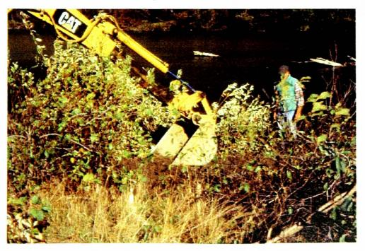
Photo 5.1. Backhoe digging trench during baffles construction, 3 Nov 1993.
