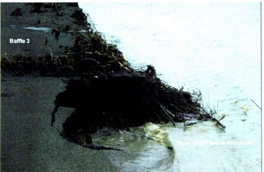
Photo 6.11. Calving bank and baffle eroding. Note wave scour below root zone occurring during flood recession 14 Jan 1995.
