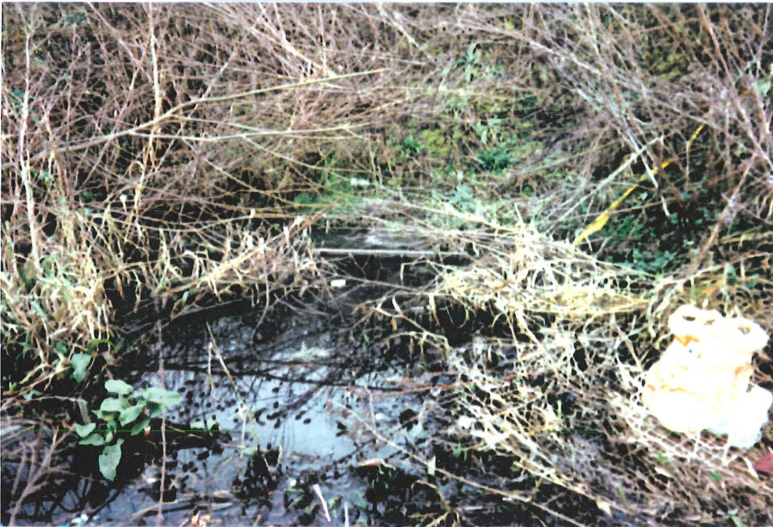
Plate 1i Submerged drain at the inlet of the wetland (Site 1).
