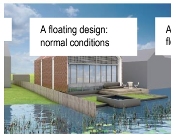
Amphibious House normal position The waterproof concrete hull of the house rests inside a fixed dock
