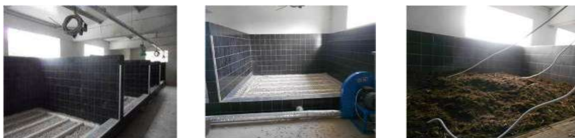
Figure 1. Aerated static pile composting system
