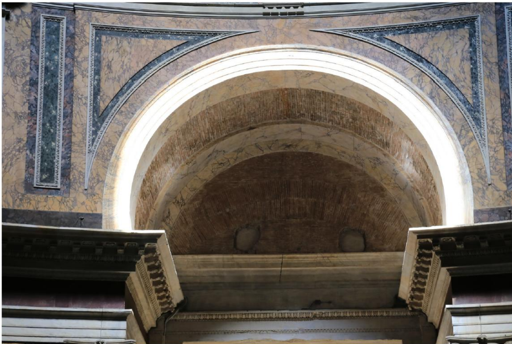
Figure 16. Detail of the Arc of Light, perfectly matching the masonry arch (photo by M. De Franceschini).
