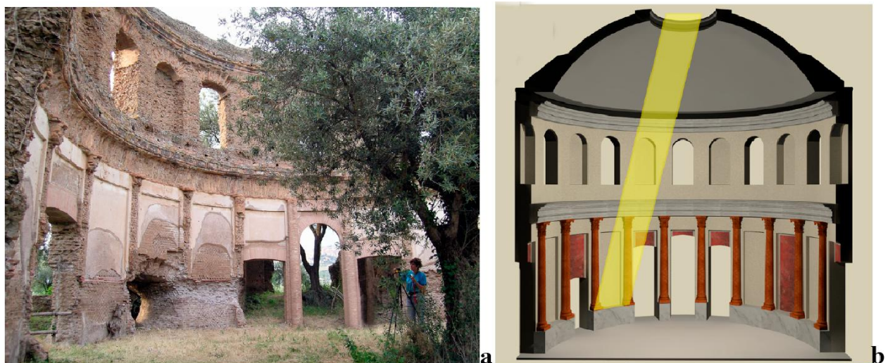
Figure 4. Temple of Apollo: a - photo of the Temple of Apollo today (only half of it is still standing); b - 3D reconstruction of the dome and of a possible illumination (drawing by Brigitta Casieri).
