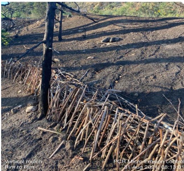
Figure 4. Terracing With On-Site Material to Control Soil Erosion Photo: Kara Dohrenwend
