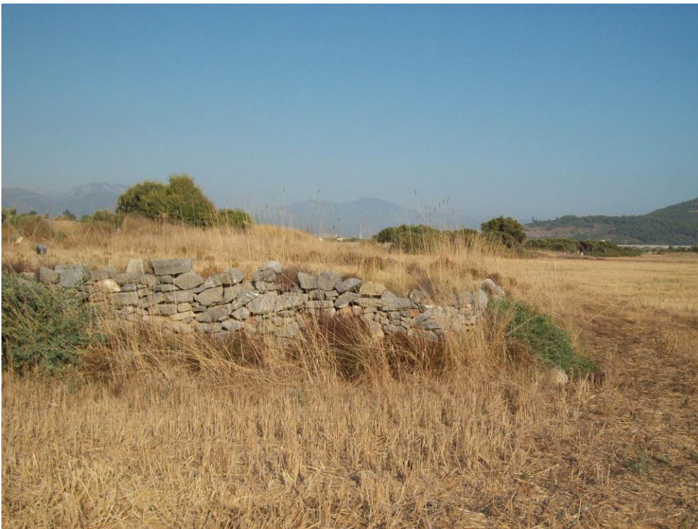
Figure 27: Retaining Wall on the East Side of the Ruined Structure at the Delice Kiln Site in 2008
