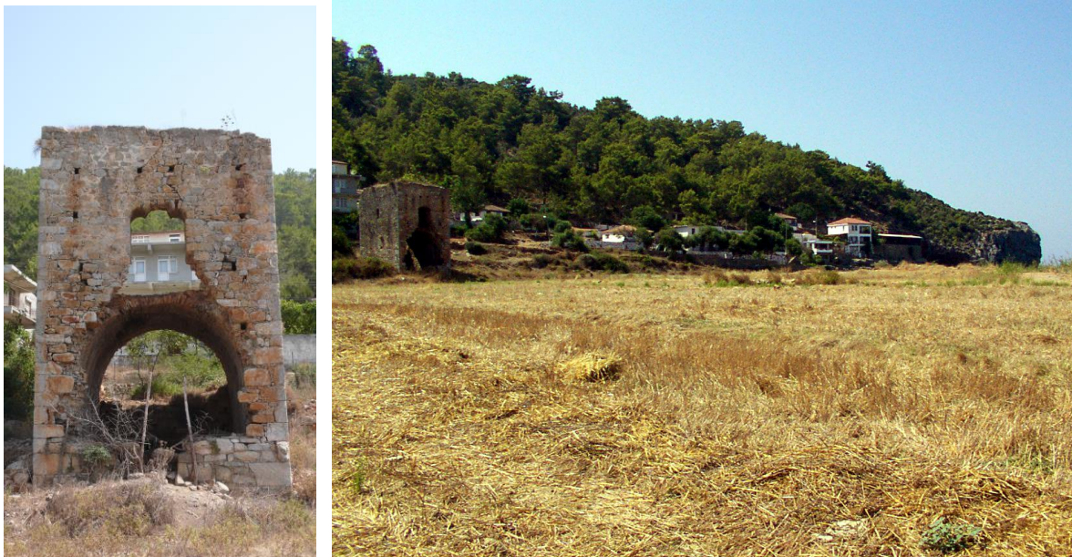
Figures 16-17: View of Roman Era Tower and Open Terrain at the Bickici Kiln Site, with Turkish Forestry Service Community in the Background
