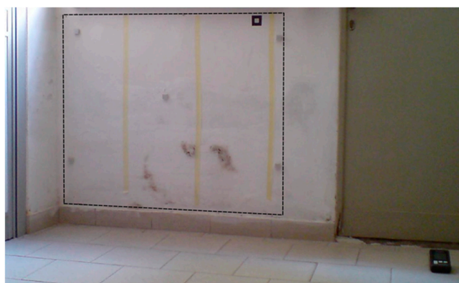
Figure 3. Plastered wall for the preliminary test with active thermography.
