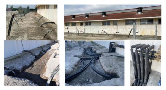
Figure 17. Realization of the BTES system: installation of the 8 BHEs and pipe connections.
