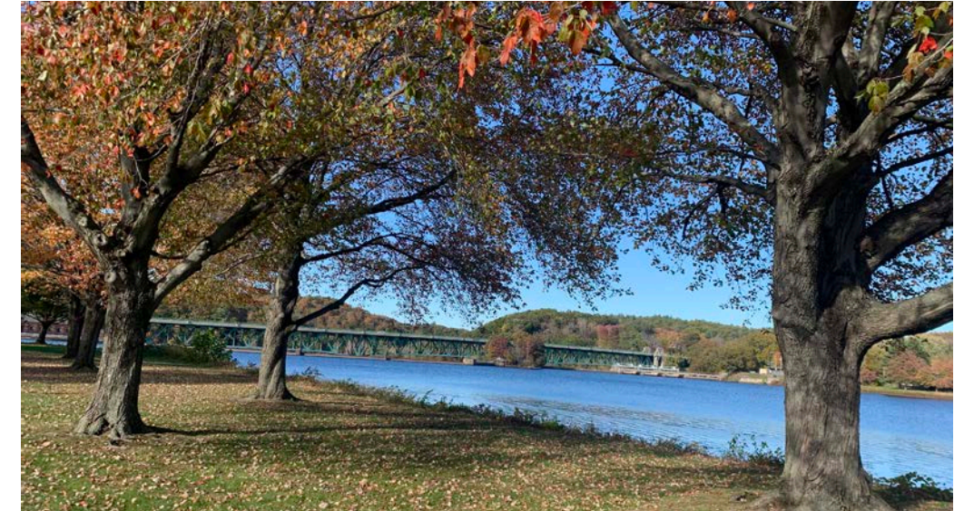
View of the Gill-Montague Bridge in the distance along the Canalside Rail Trail
