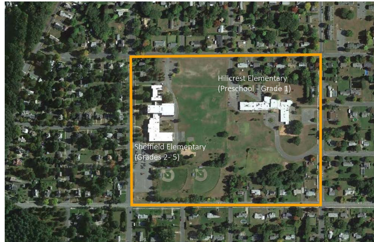
Aerial view of existing project site
