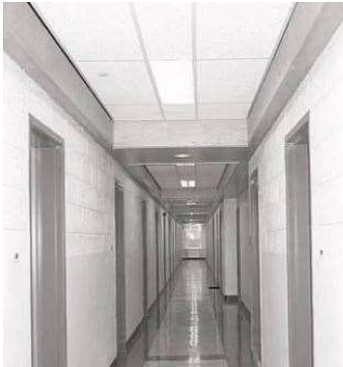
Figure 34: North-south first-floor corridor facing to the north.
