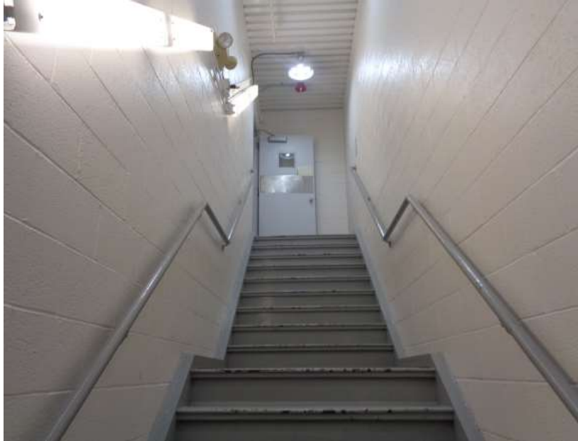
Figure 39: Interior exit access stairway from the lunchroom.
