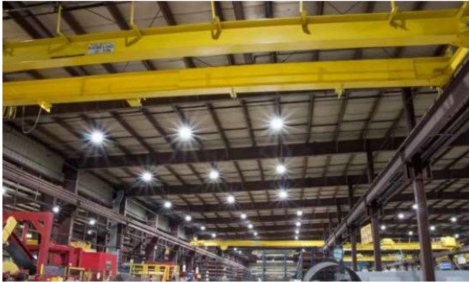
Figure 53: Main high bay in PNNRA-517.
