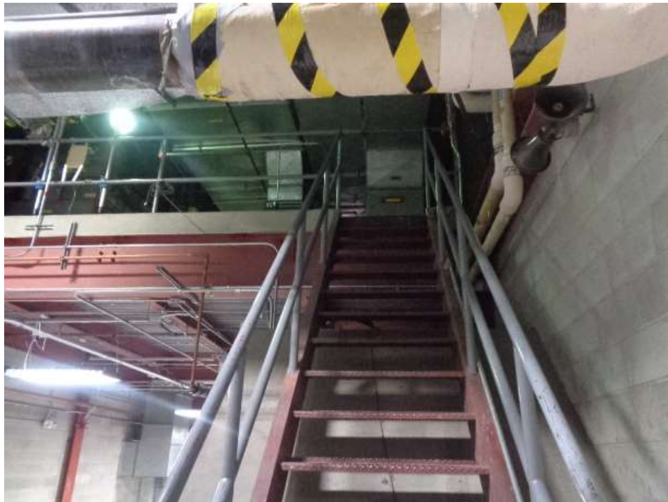
Figure 55: Mezzanine above the fan room.
