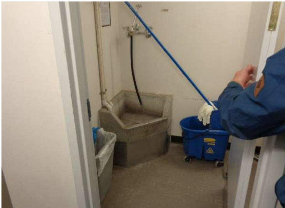
Figure 33: Janitors' closet behind door 107.
