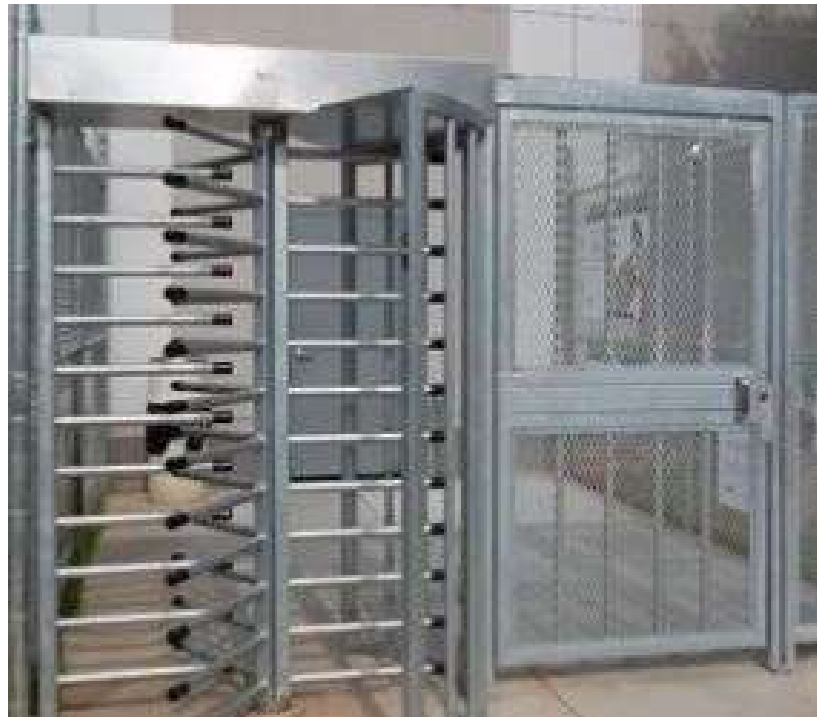
Figure 9: Near the SFPF breakroom. Notice that adjacent Door provides egress.
