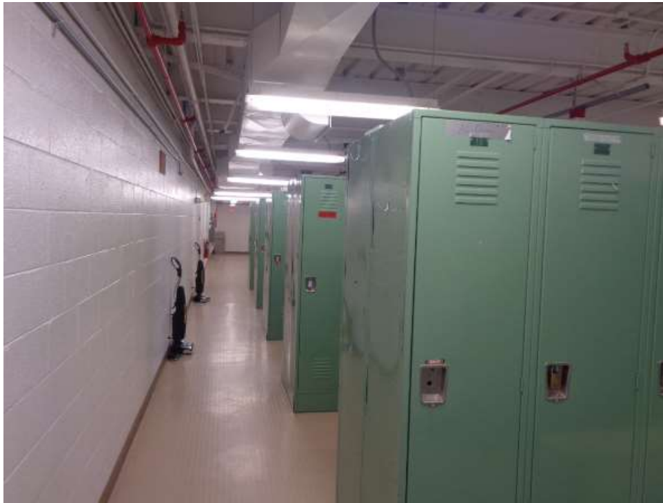
Figure 37: Mens' locker room near door 112A.
