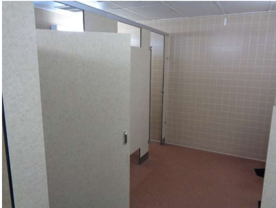
Figure 35: First-floor bathroom behind door 110.
