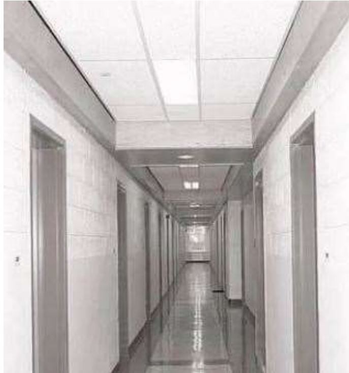
Figure 7: The fire door next to breakroom (Balloon 78 in Figure 72).
