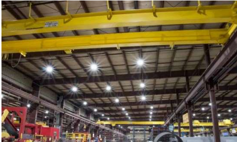
Figure 57: Door 52 waste processing area just to the south of the main PNNRA-517 high bay.
