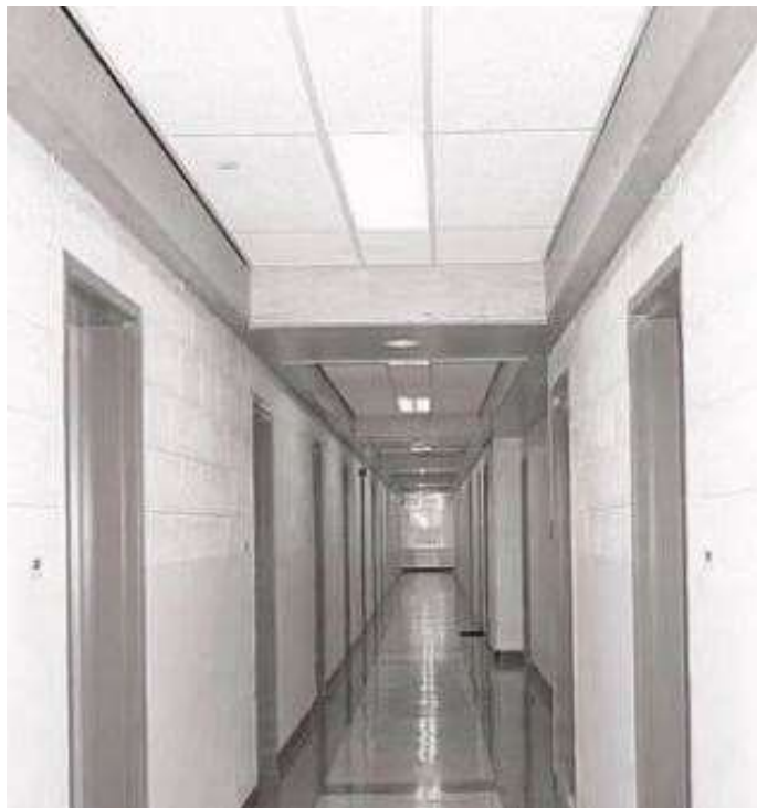
Figure 16: Corridor inside of Door N-26U on the north side of the ACME Building.
