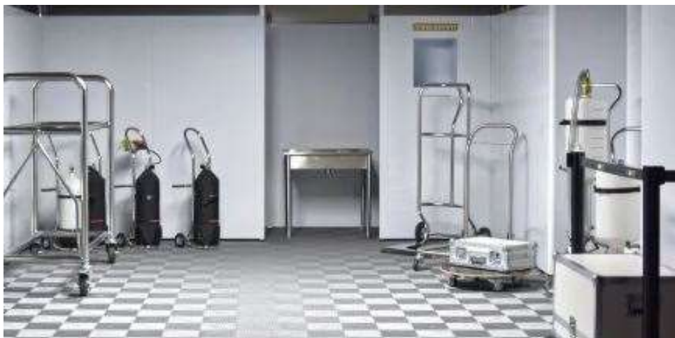
Figure 62: Aisle within the elevator equipment access pit in PNNRA-438.
