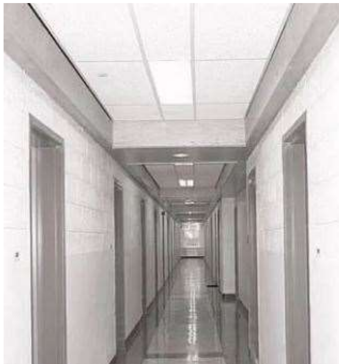
Figure 46: East hallway (205) on 2 nd floor that leads to the exterior exit stairway.
