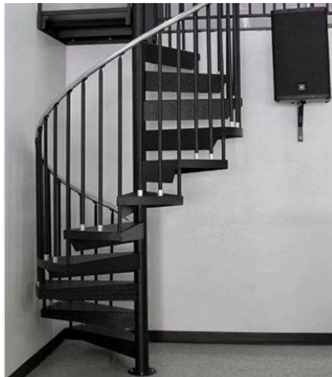
Figure 14: Spiral staircase from the Facility Manager's office, which leads to the Fan Room.
