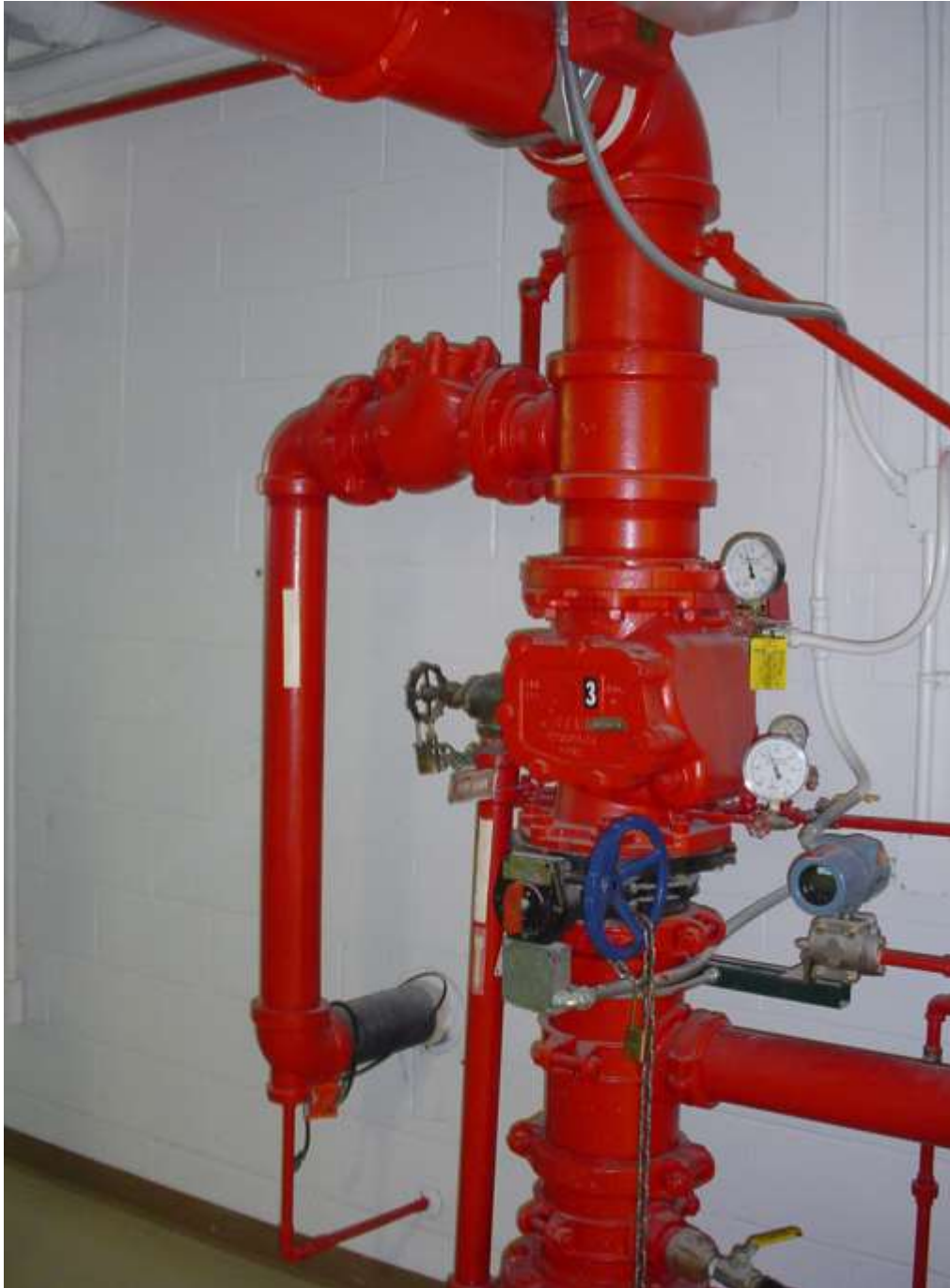
Figure 128: Riser for System 3.
