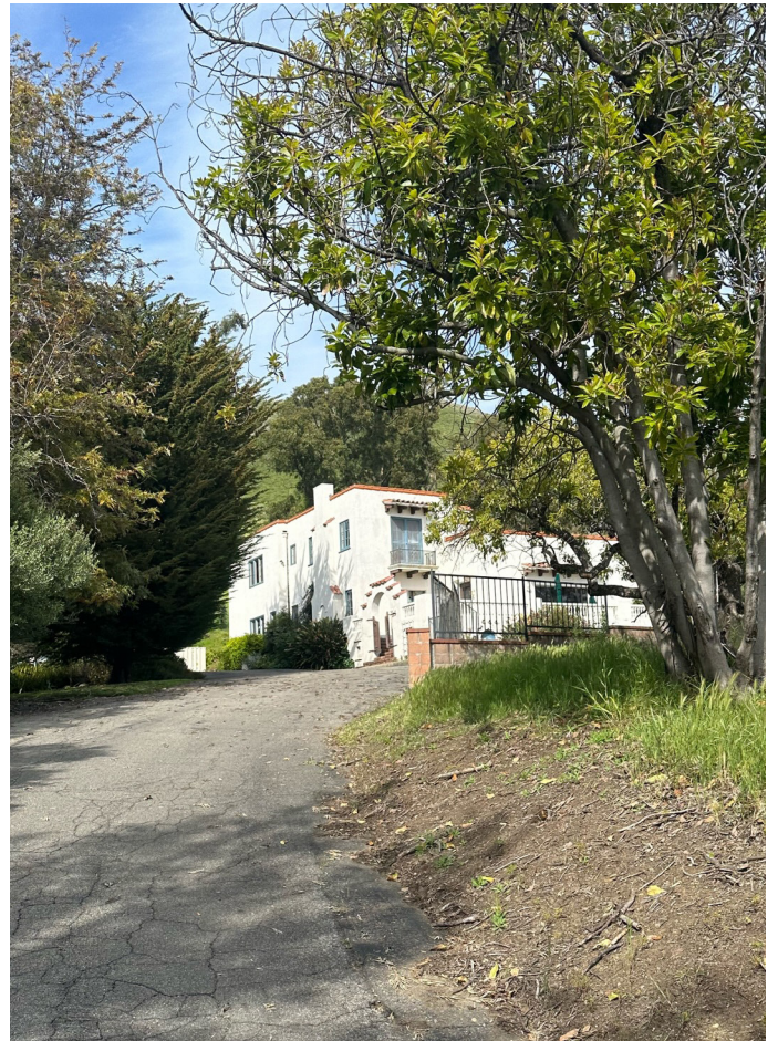
Avila Residence from Site Visit 4/17/23
