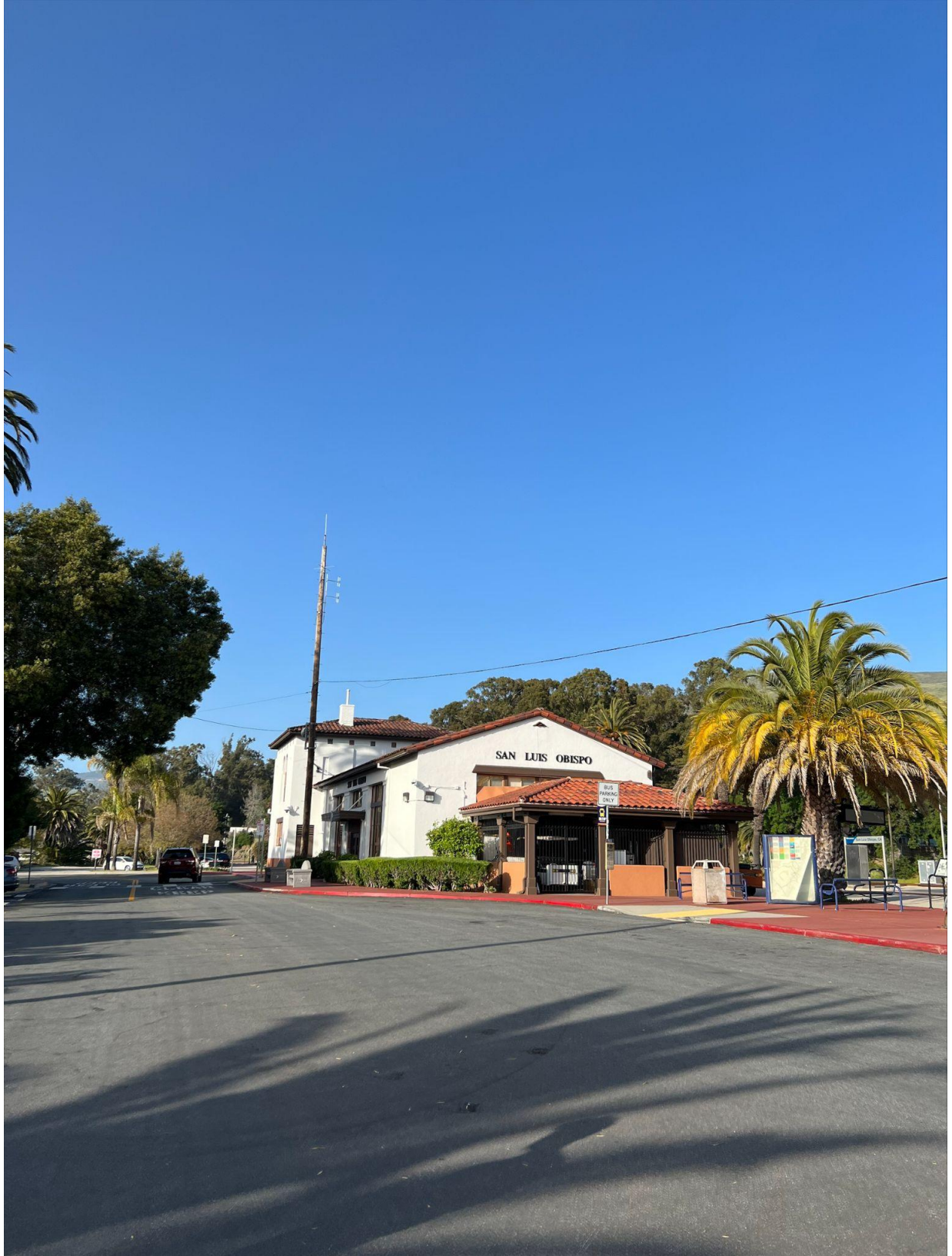
Image/Figure 11 - View of the train station, looking north (2)
