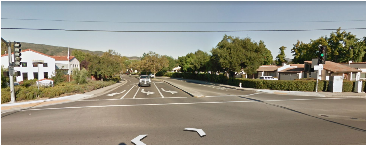
Figure 1-4: Intersection of Los Osos Valley Road and S. Higuera St.
