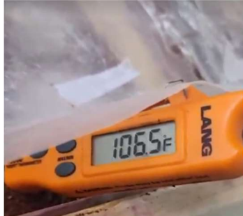
Figure 9 Temperature Probe Showing a 106.5° F Brick
