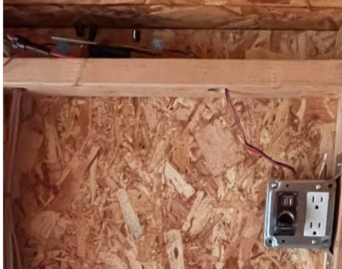
Figure 5.7 12-Volt DC system Dual USB Power Outlet and 15A - 125V Heavy Duty
