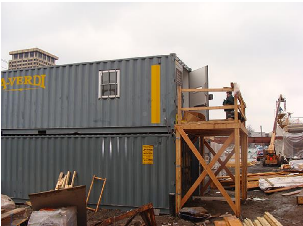
Figure 4: A-Verdi- Jobsite Trailer constructed out of shipping containers.
