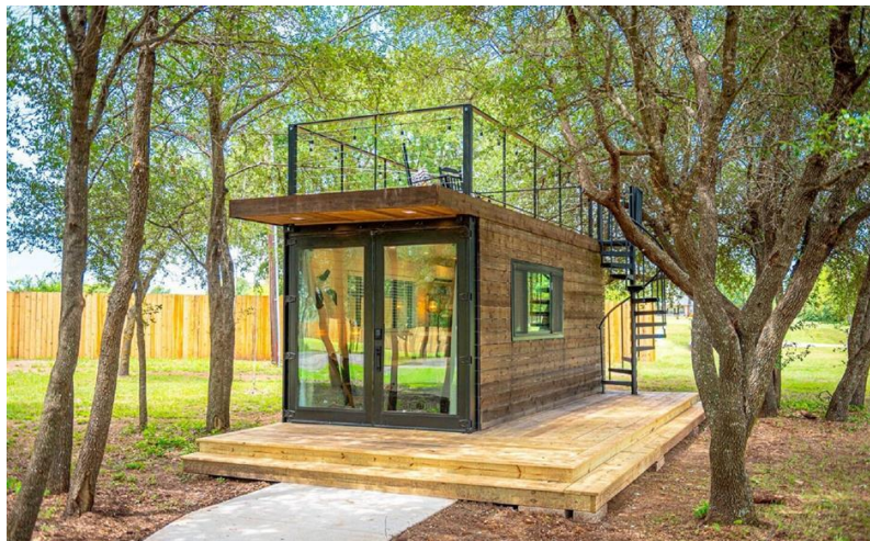
Figure 2: Homes Beautiful- Single 20-foot prefabricated shipping container home
