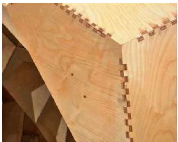
Figure 12 Interlocking Finger Joints: ICD/ITKE 2011 Research Pavilion
