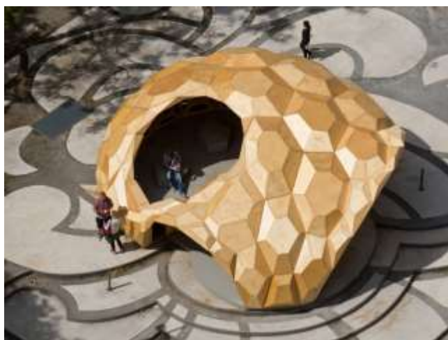
Figure 11 Interlocking Finger Joints: ICD/ITKE 2011 Research Pavilion
