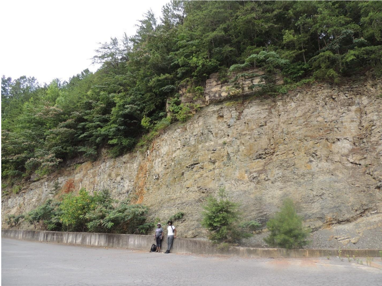
Figure 4.2 Studied section of the AL-1 outcrop, located behind United Grocery Store in Fort Payne, Alabama.
