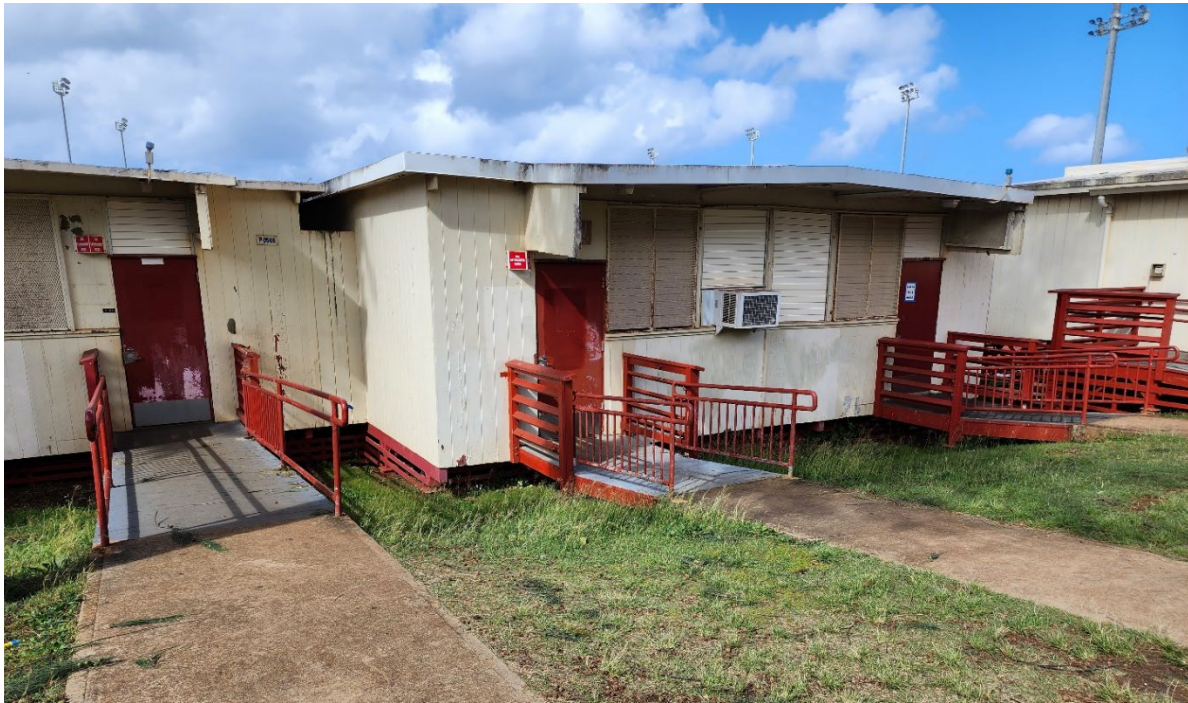
Figure 28. Kahuku High School Classrooms.
