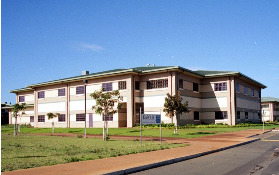
Figure 35. Kapolei High School Classrooms.
