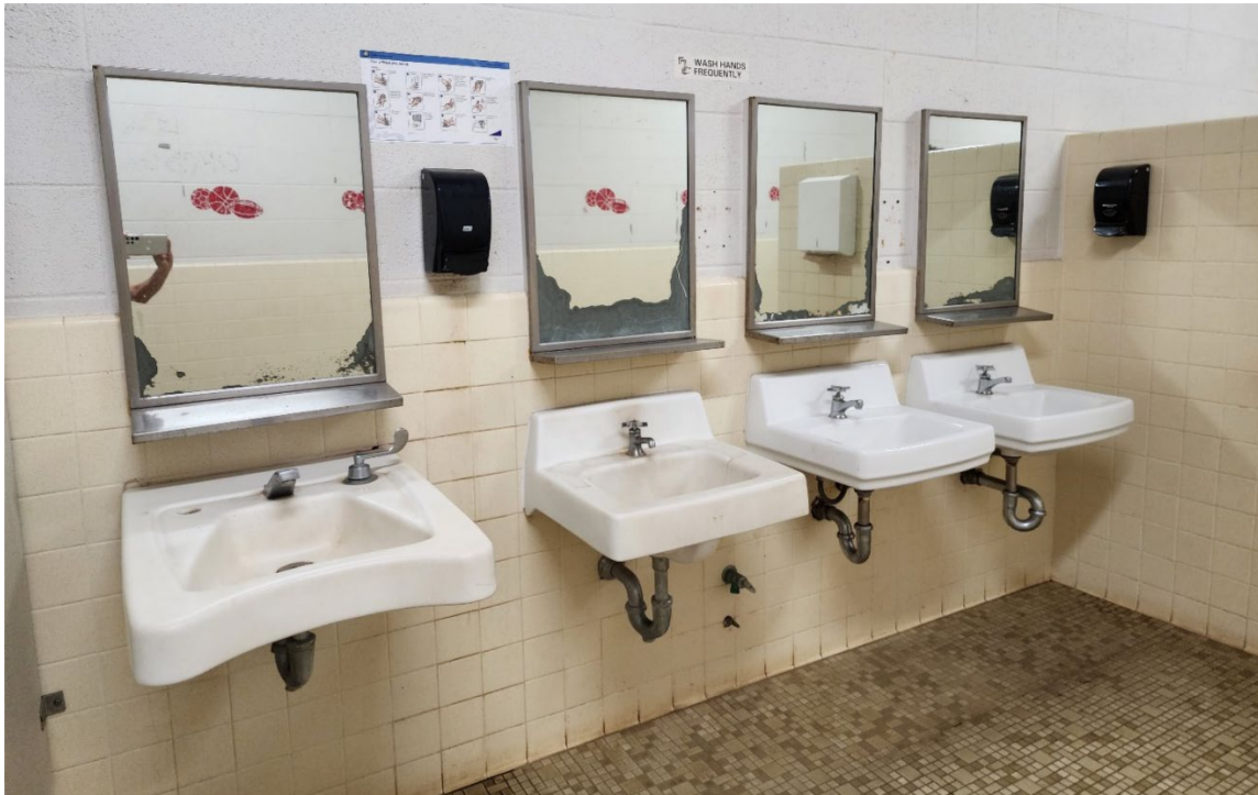
Figure 32. Kahuku High School Restroom.
