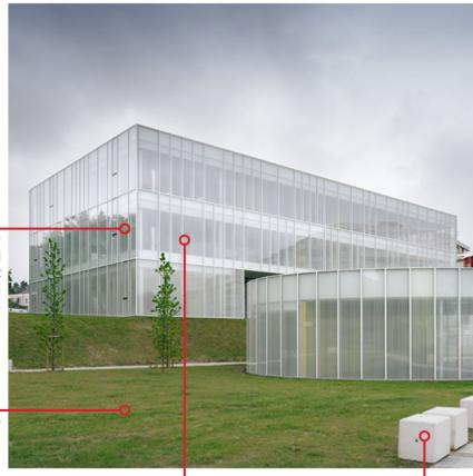
Translucent glass provide privacy to the building during the day and becomes complete transparent during night due to difference in illumination from inside versus lighting of the exterior surrounding.
