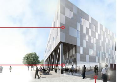
Window install flush to floor increases large view port to the surround landscape, rainwater will penetrate without proper waterproofing during construction. White mesh balustrades to increase semi-visual transparency in transitional spaces with the entire design intent to replicate Greek amphitheaters.
