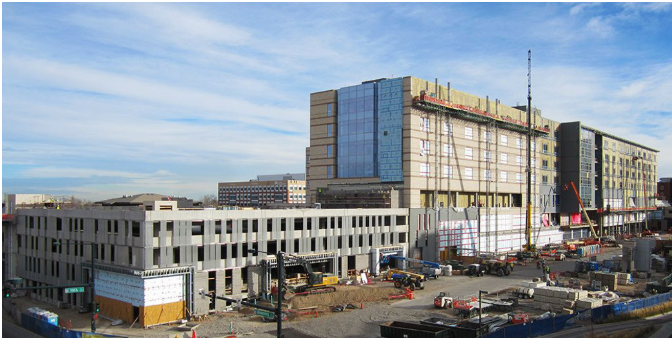
Figure 40 | St. Joseph Construction
