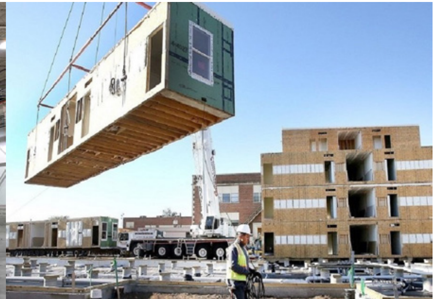
Figure 30 | Ellis Module Crane
