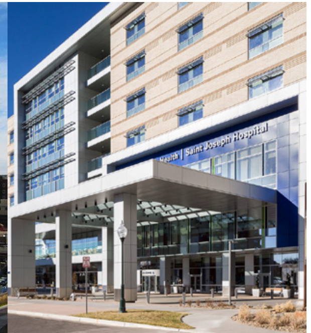
Figure 41 | St. Joseph Entrance
