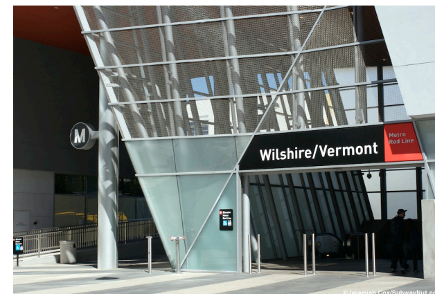
Figure 2.8 - W.V. Metro Station Entrance
