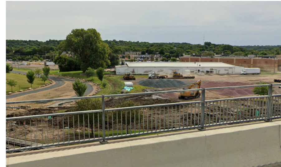
Figure 2.30 - Site View 1 North West
