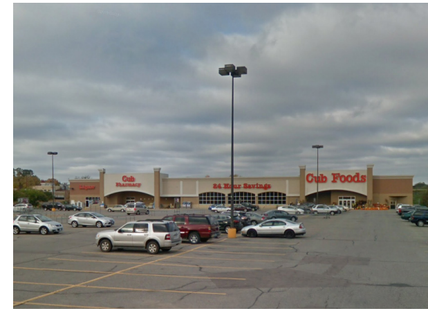
Figure 2.38 - Analysis of Notable Building Surrounding Site
