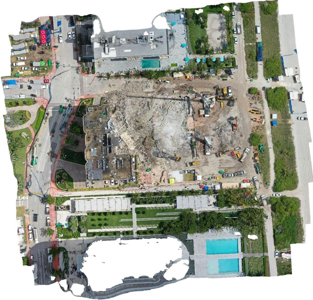
Figure 1.1: Orthomosaic of Surfside Condominium Collapse
