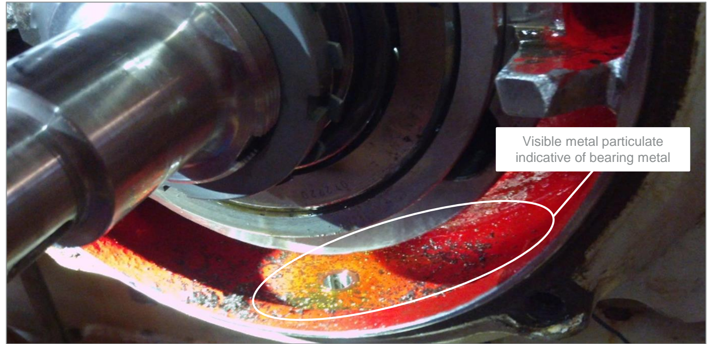
Figure 9: Pump NDE Bearing Inspection showing metal particulate.
