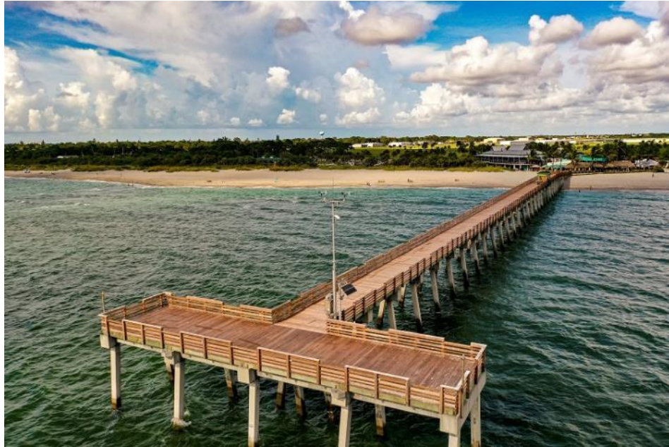
Figure 4. Pier Made of Timber
