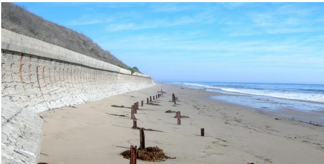
Figure 5. Concrete Sea Wall
