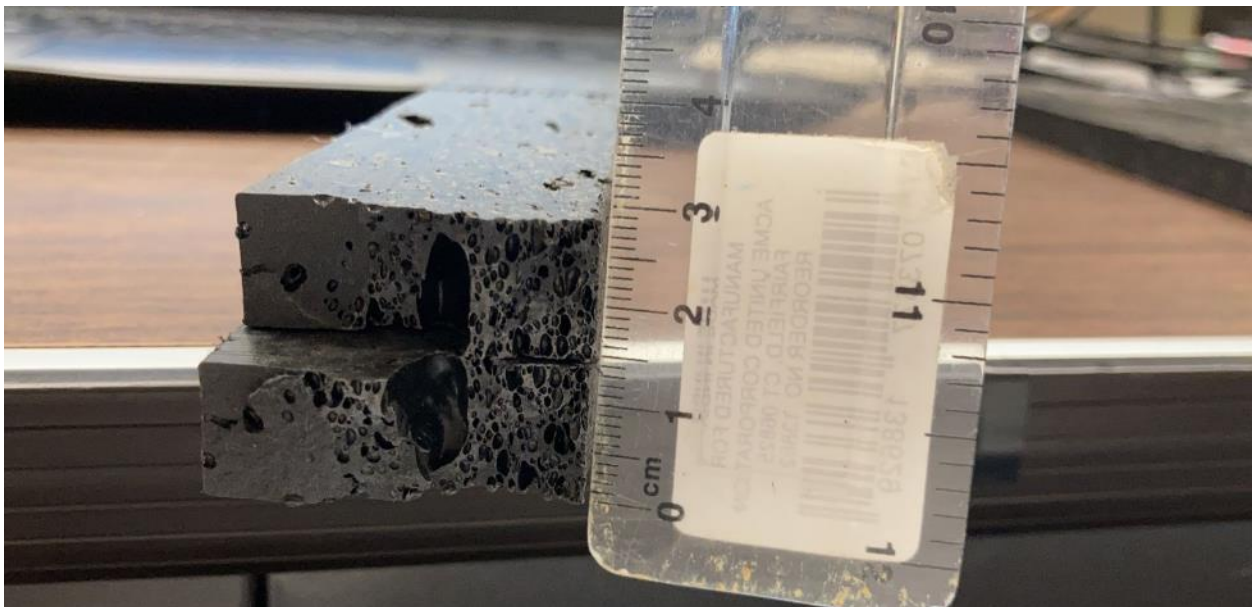
Figure 90. Detailed View of Damaged Area of Sample D1_2
