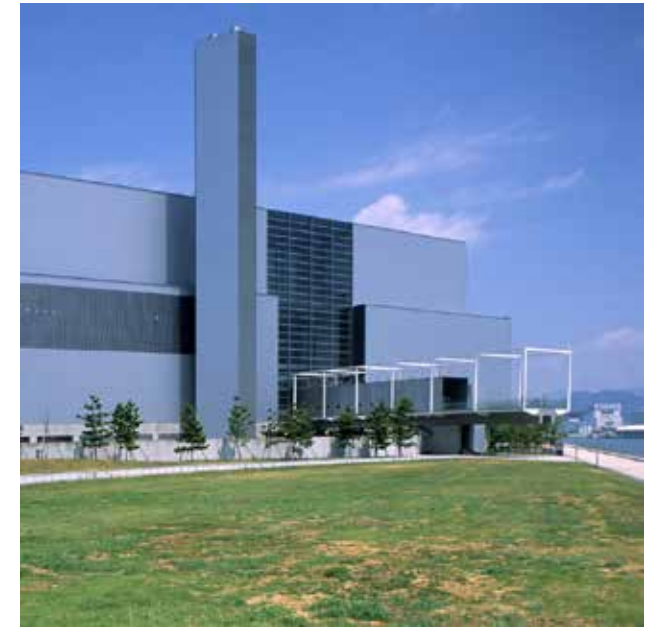
Figure 9. Naka Incineration Plant, Photo by Larry Speck
